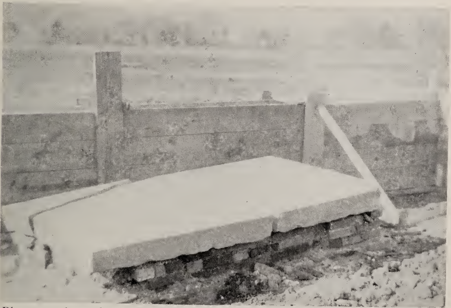
Photograph made during the restoration work in 1923
